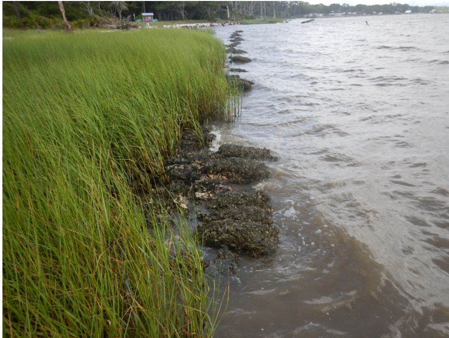
Photograph C6.1 Oyster Breakwater, Cat Point in the Florida Panhandle
