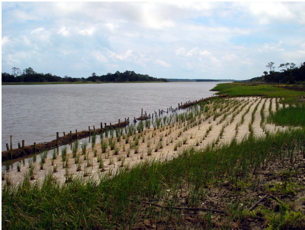
Photograph C6.2 Marsh Restoration in St. Johns County, FL
