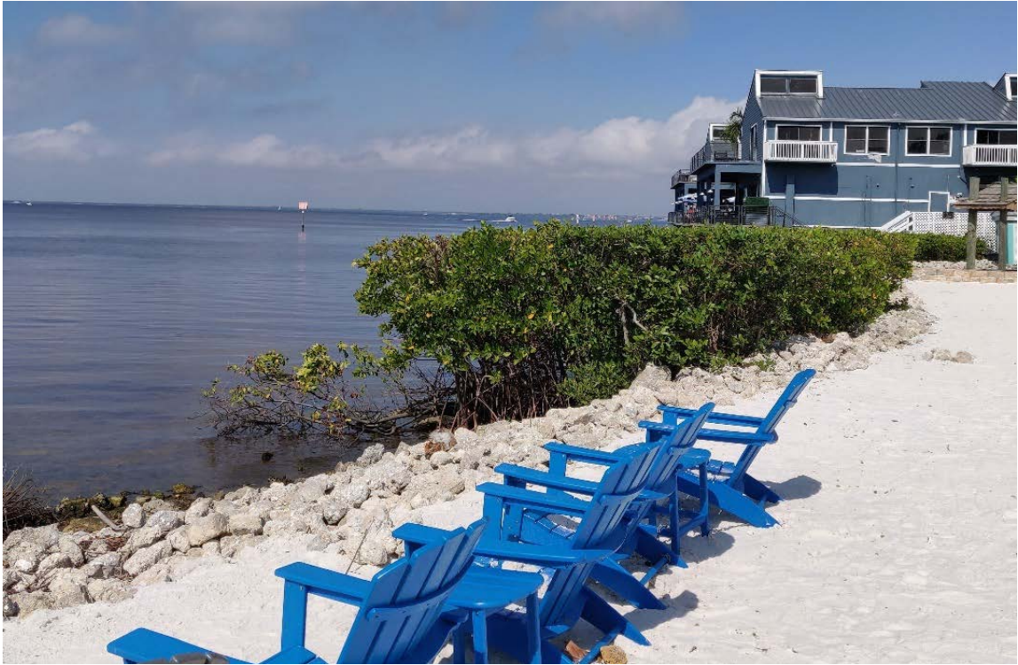
Photograph C2.1 Mangrove Living Shoreline, February 2019
