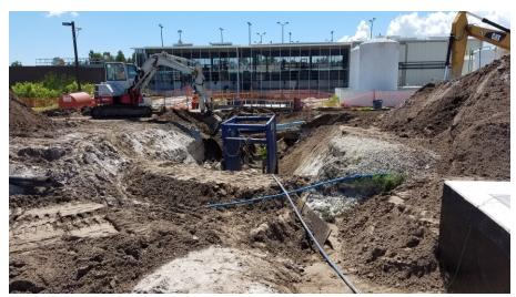
Connecting the pipework to tie the blend basin into the storage tanks.
