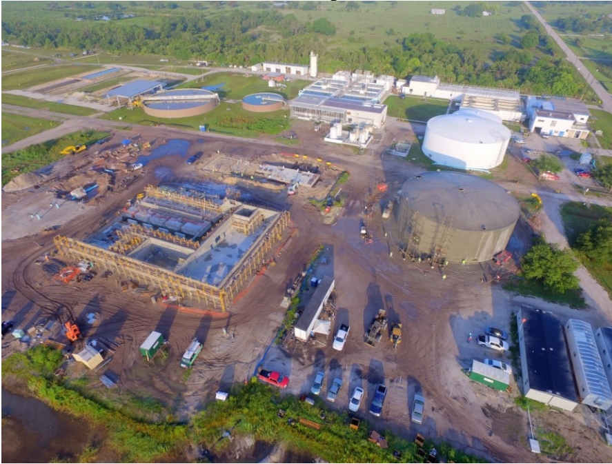
Week 49- Overview of plant site.
