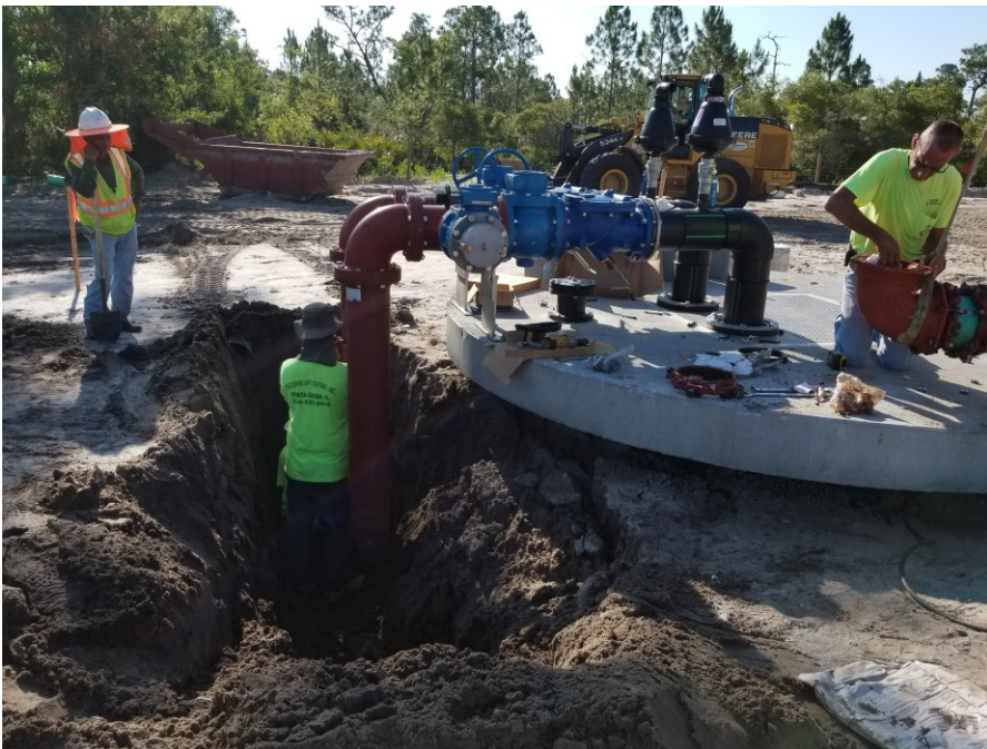
Wastewater Treatment Plant 20 inch Force Main Replacement Project
