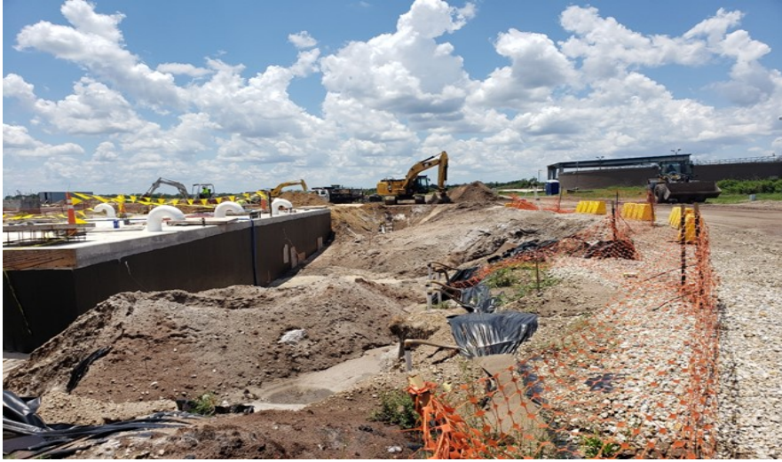
Week 48 - Backfilling around blend basin.
