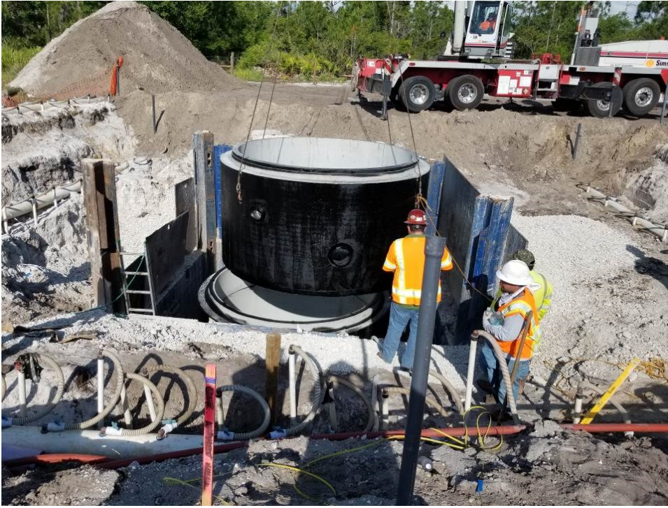
Photo of wet well construction
