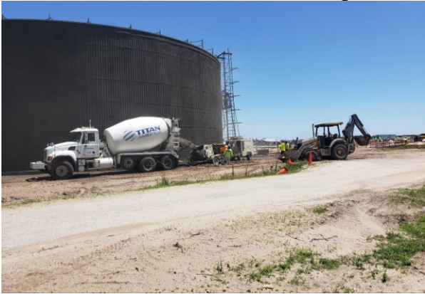
Week 43- Continuing work on the new two million gallon storage tank.
