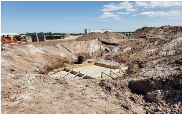
Week 43 – Starting work on the degasifier.
