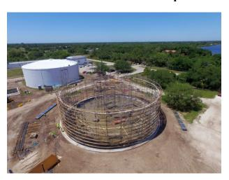
Week 42- Scaffolding set up for the forming of the new 2 million gallon storage tank
