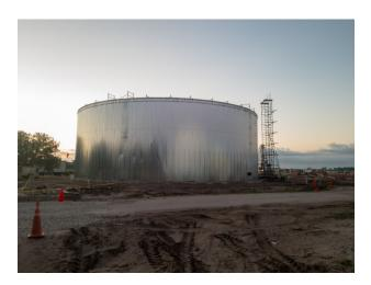
Week 42- Forming panels installed for the new 2 million gallon storage tank.
