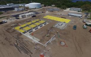
Week 41- Installing the pipeline to connect the blend basin to the existing 2.0 million gallon tank.
