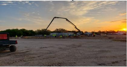
Week 40: Placing the base slab of the 2.0 Million Gallon Storage Tank.
