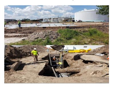
Week 39- Started construction on the pipeline to connect the existing 2.0 Million Gallon tank to the blend basin.
