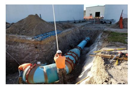
Week 37 – Installing the water line to connect the new and existing 2.0 million gallon finished water tanks together.
