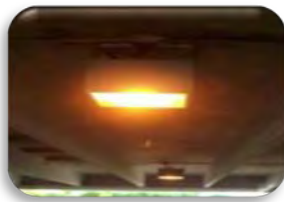
High Pressure Sodium Light Fixture
