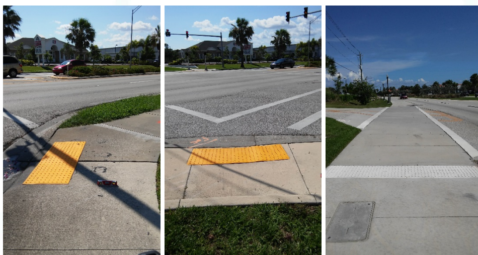
Figure 4-2 - Curb ramps and detectable warning surfaces along the multi-use trail.
