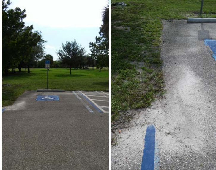
Figure 4-1 – Existing Accessible Parking Space in the East Lot
