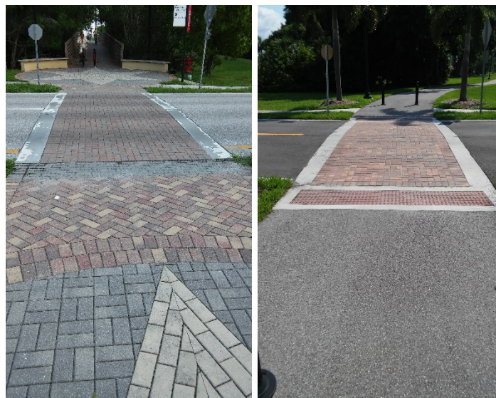
Figure 4-1 - Detectable warning surfaces along the multi-use trail.
