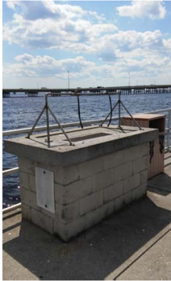
Figure 4-14 – Fish Cleaning Station
