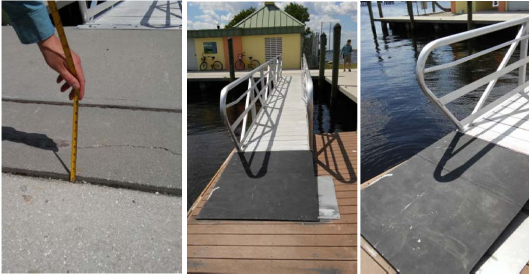
Figure 4-12 – Gangway and Transition Plate Leading to Single Floating Boat Slips
