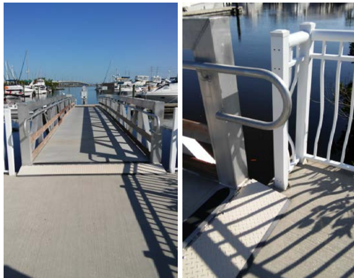
Figure 4-8 – Top of Gangway to Boat Slips
