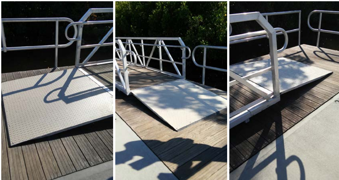
Figure 4-9 – Gangway and Transition Plates at Ends of Floating Dock along Harborwalk
