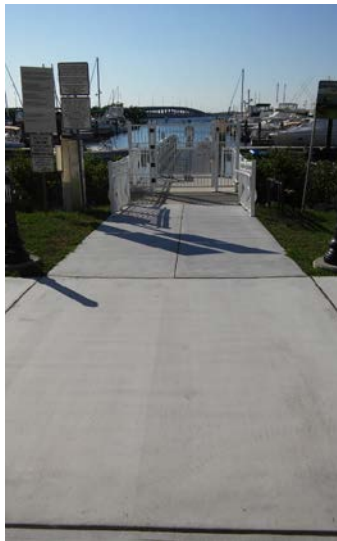
Figure 4-7 – Ramp leading to Gate
