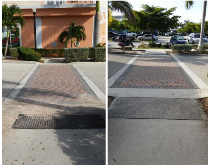
Figure 4-4 – East Crosswalk and Path to Leased Facility
