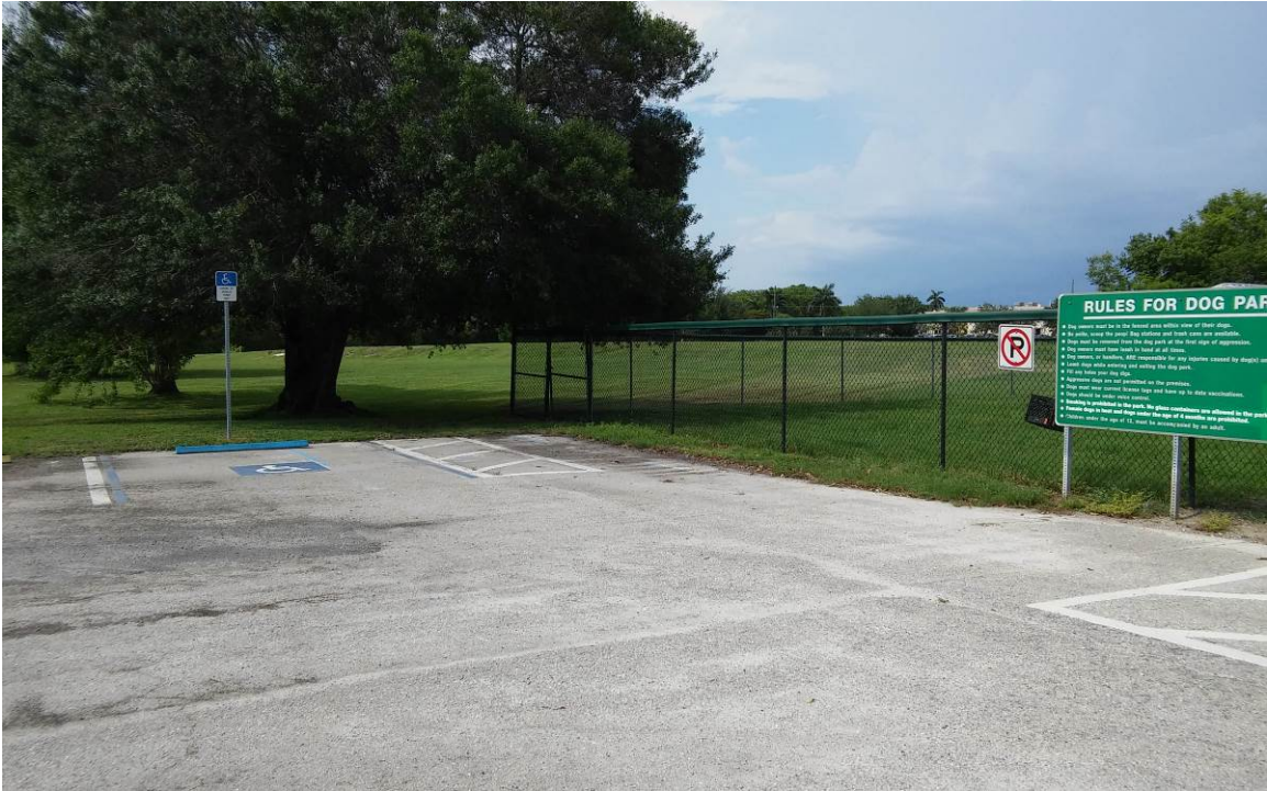
Figure 4-3 – Access aisle and accessible route
