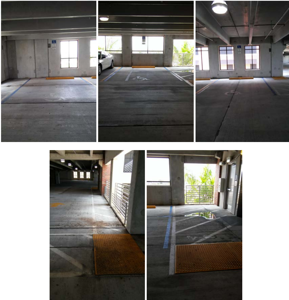
Figure 4-2 – 3 rd Floor Parking Area
