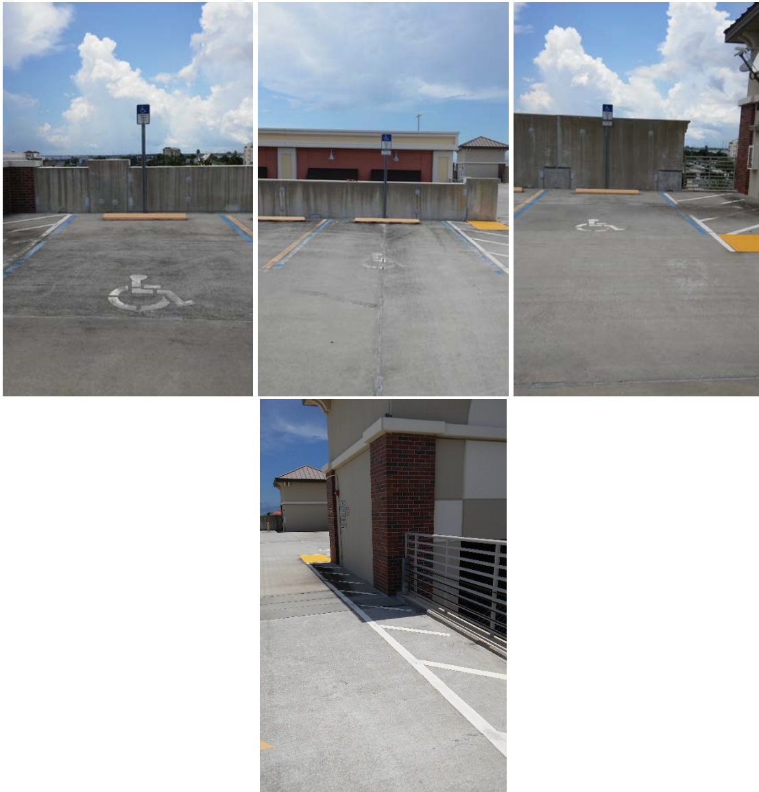
Figure 4-3 – 4 th Floor Parking Area
