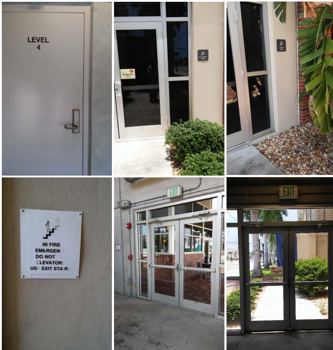
Figure 4-4 – Examples of doorways without ADA compliant signage.
