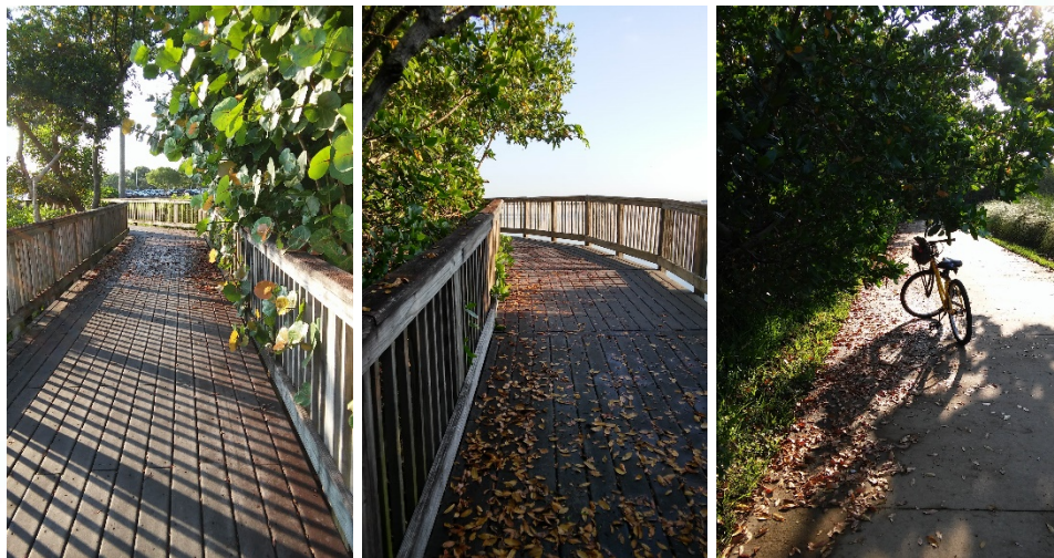
Figure 4-2 – Low hanging tree branches
