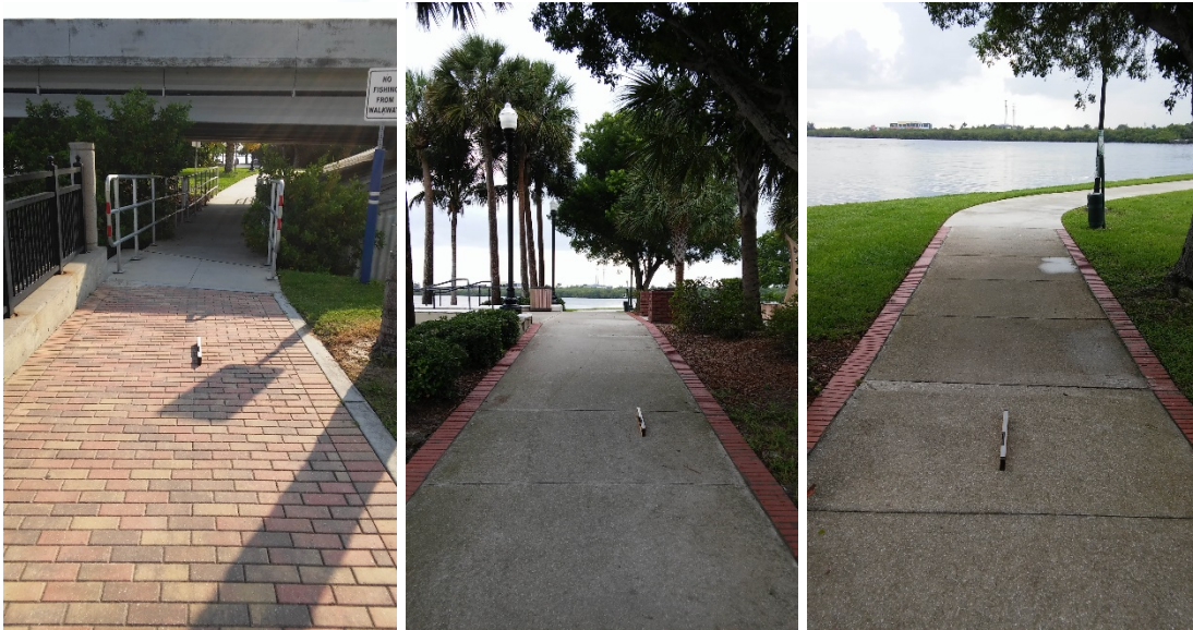
Figure 4-5 – Select locations with non-compliant cross slopes.
