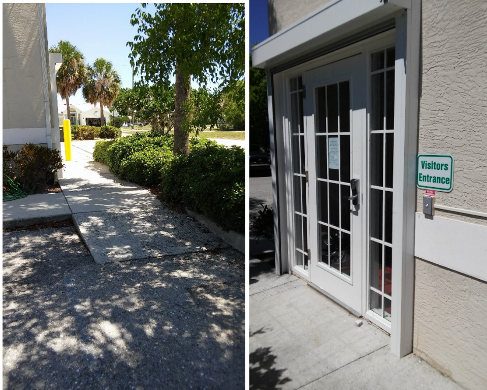
Figure 4-2 – Curb Ramp and Public Entrance
