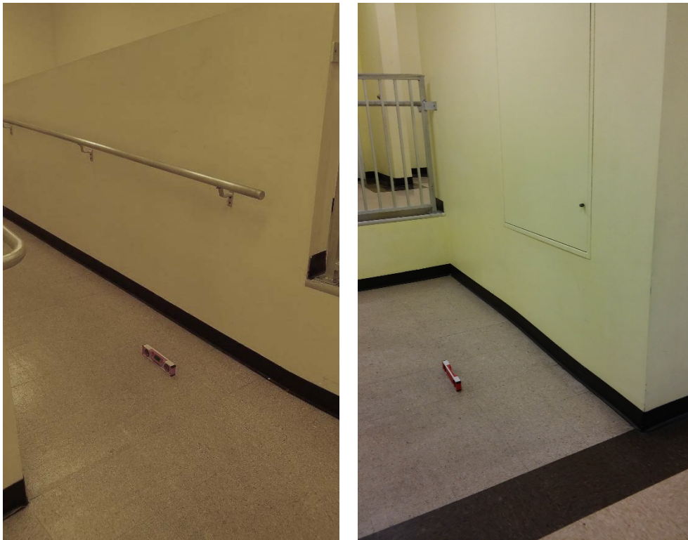
Figure 4-10 – Interior Ramp and Handrails
