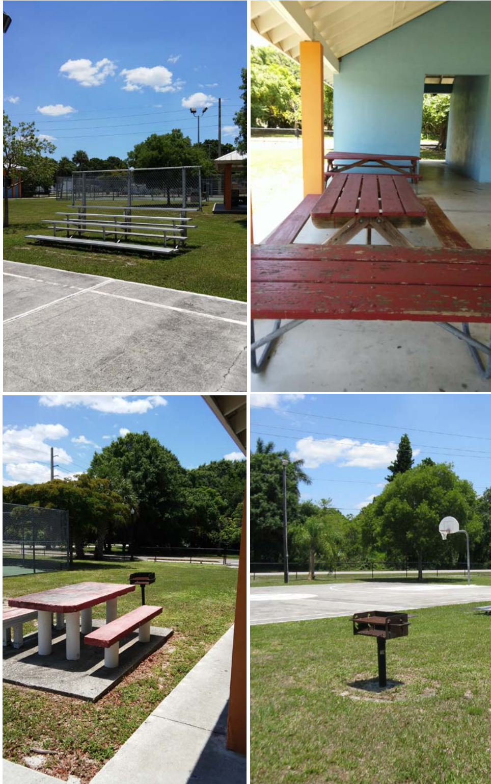
Figure 4-5 – Non accessible outdoor elements
