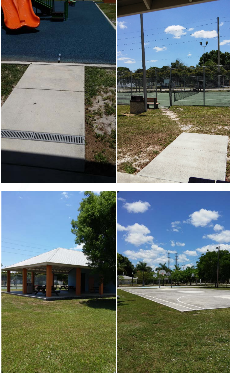
Figure 4-4 – Non accessible outdoor elements
