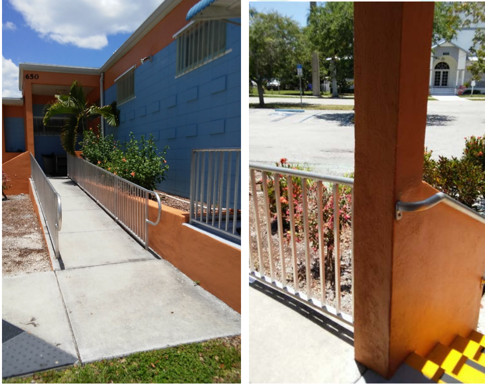
Figure 4-3 – Ramp leading to the raised public entrance.
