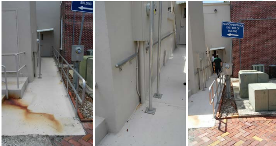
Figure 4-5 – Ramp to Rear Entrance
