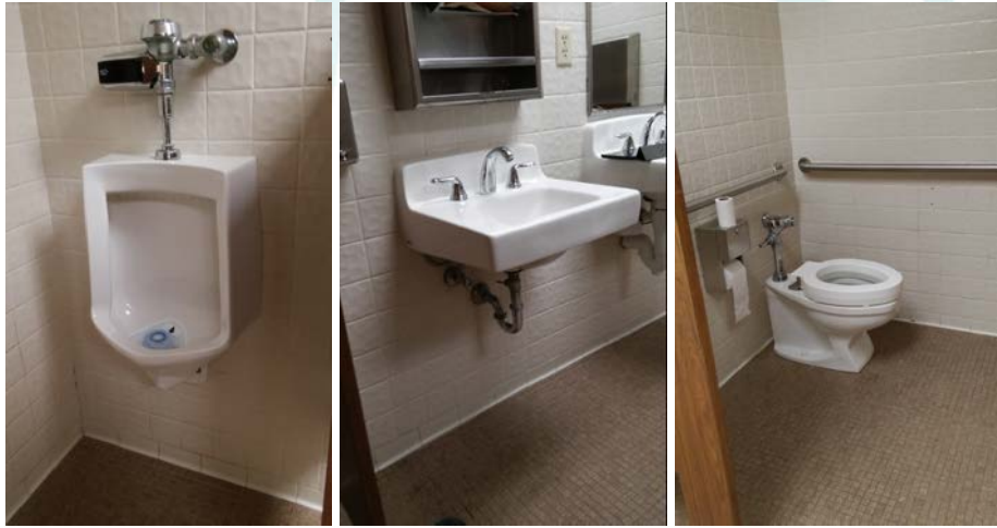
Figure 4-10 – First Floor Men's Room
