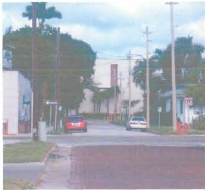
Existing South Side of Auditorium
