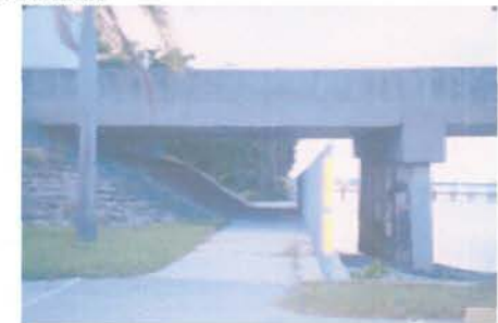
Existing Bridge Underpass
