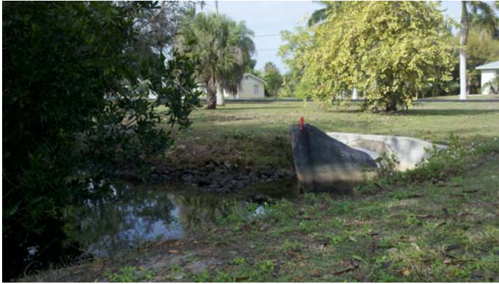
TIDAL FLAP ON STORMDRAIN PITFALL IN A TIDAL CANAL
