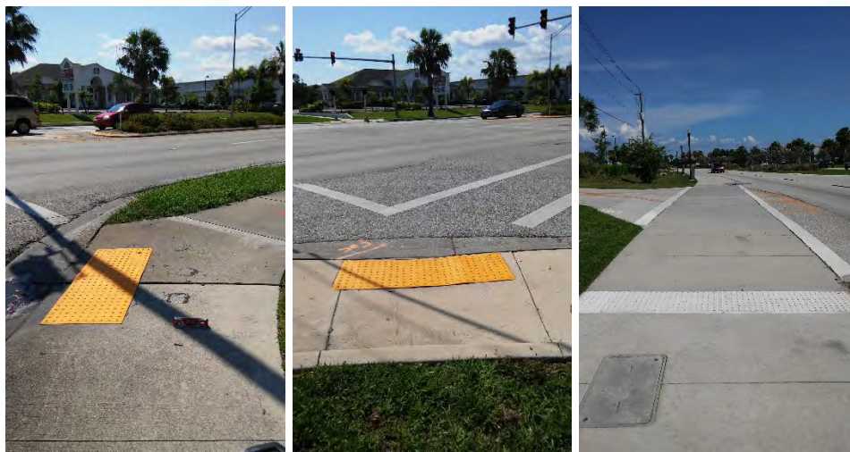
Figure 4-1 - Curb ramps and detectable warning surfaces along the multi-use trail.
