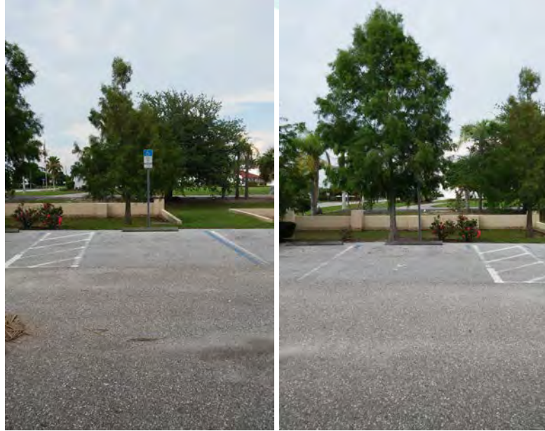
Figure 4-1 – Existing accessible parking spaces
