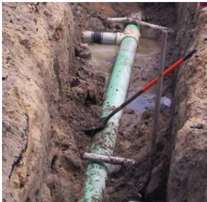
Gravity Sewer Replacement Project
