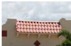
Barrel Tile Roof
