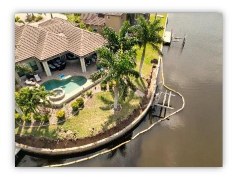
• Establishing sod after seawall replacement – Placing the sod is the final phase of seawall replacement construction. As per the City ordinance, property owners are responsible for establishing the sod after it has been placed and the City will not reimburse the owners for their water usage.
