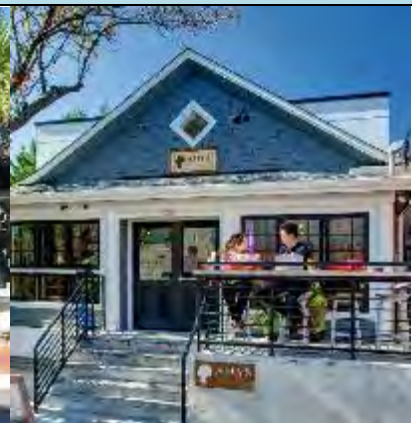
House to Café Conversion in Seattle, WA
