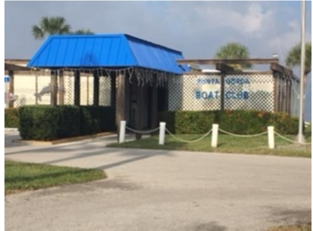
Figure 2: Boat Club Building constructed in 1962, the building has a total floor area of 4,230 square feet.
