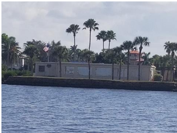
Figure 4: Boat Club as seen from Charlotte Harbor. The land lease for this facility expires in 2021, after that it is renewable in 1-year increments with a 30-day cancellation clause.
