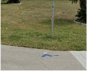
the base of the "V" indicating how far from the base of the "V" the valve lid is. Needless to say, Ed's idea has saved many hours searching for a shut off valves enabling crews to isolate water main breaks more effectively. Thanks Ed!
