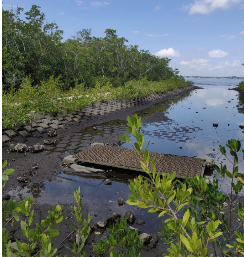
Photograph 4.6 Drainage Culvert along Punta Gorda’s HarborWalk
