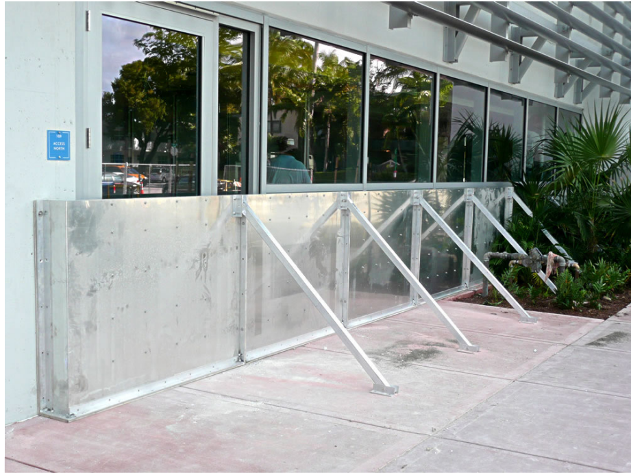
Photograph 4.4 Temporary Flood Barrier Protecting Building Entryway
