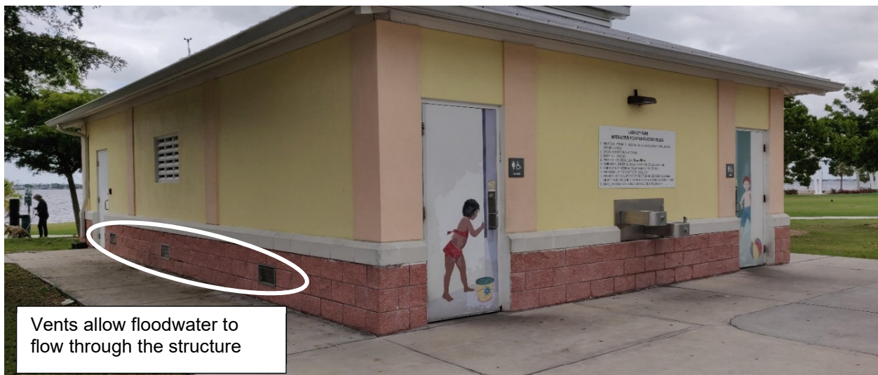
Photograph 4.1 Wet Floodproofing (Accommodate Strategy) at Lashley Park
