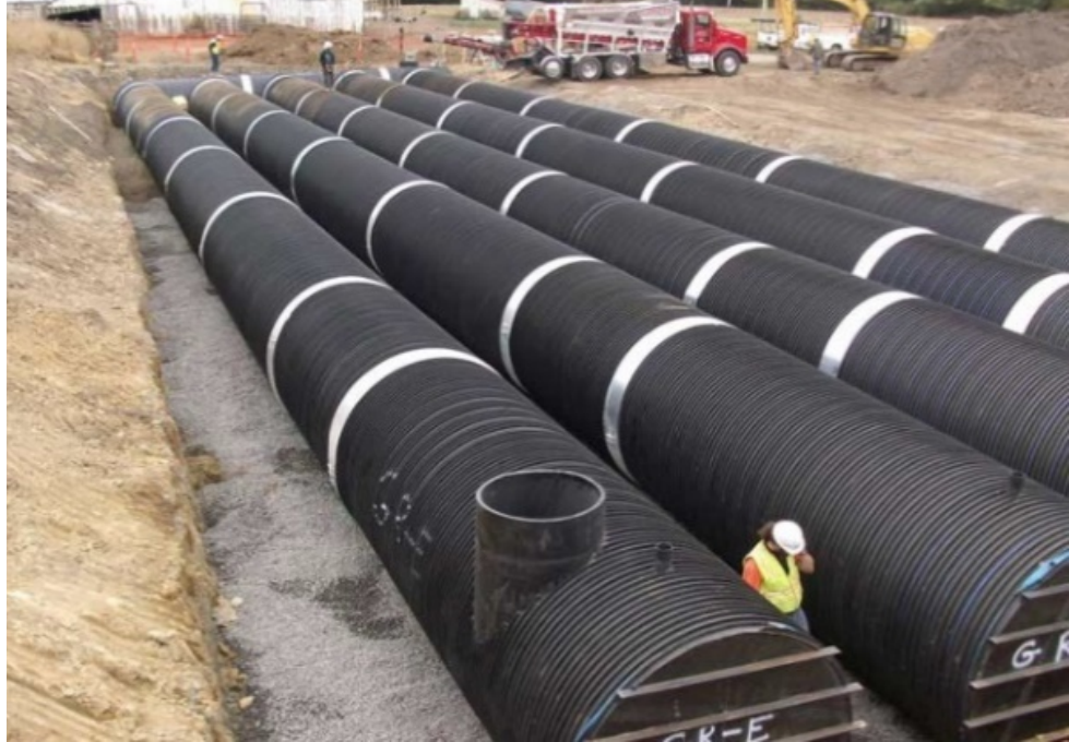
Photograph 4.5 Storage Tanks for Excess Runoff ( www.conteches.com )
