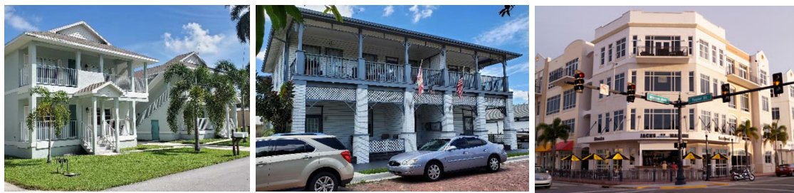
Figure 1.1 – Existing Development in Punta Gorda (from left to right): Duplexes: 22 DUA, Small Multifamily: 33 DUA, Mixed-Use Multifamily: 17 DUA (currently, there is only residential on the fourth floor, though density would be roughly 32 DUA if the second and third floors were also condo apartments instead of offices)
