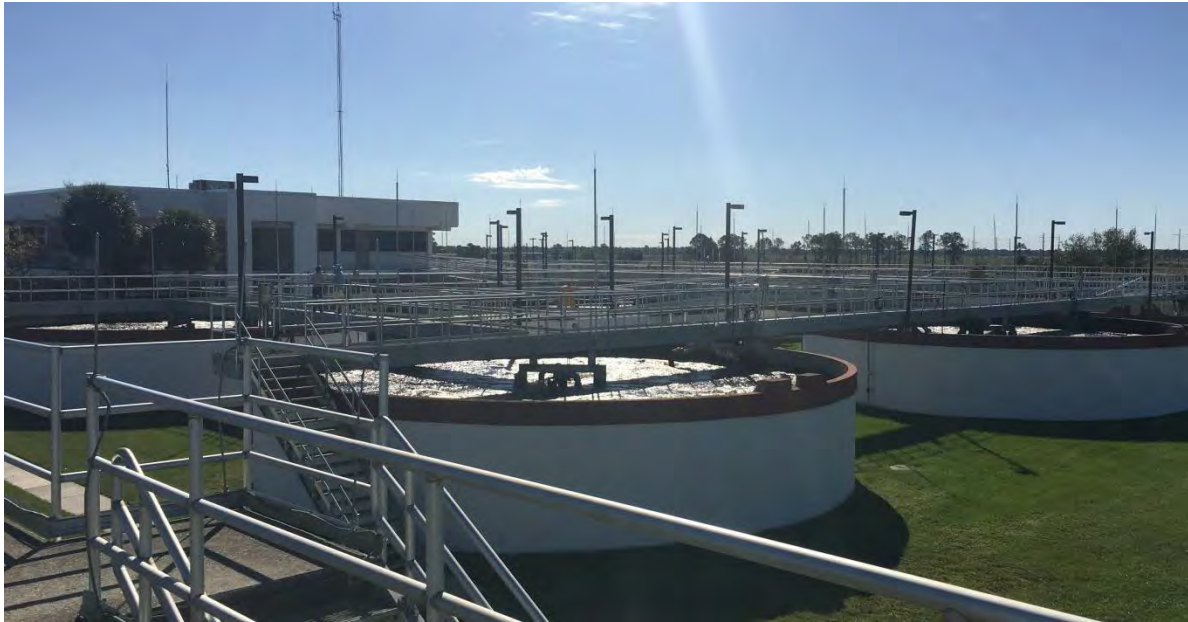
Figure 5-4 Punta Gorda WWTP – Aeration Tanks
