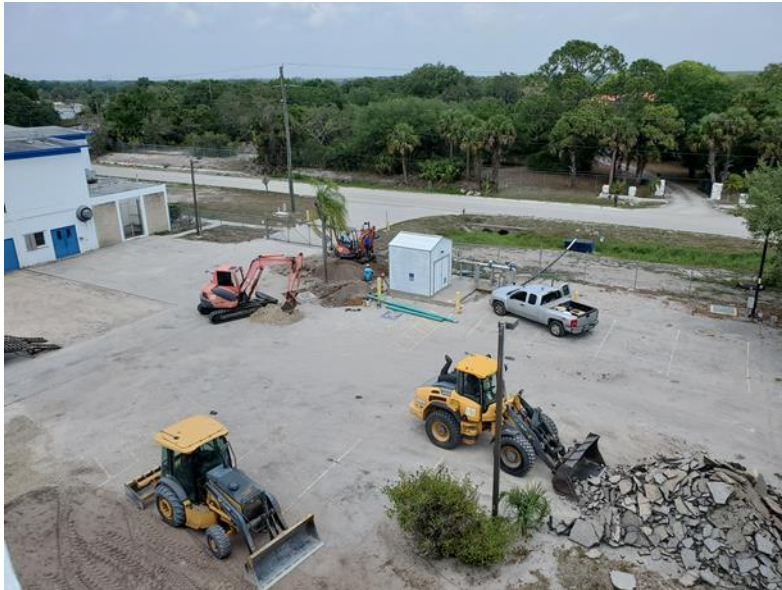
Week 93- Improvements to drainage at existing surface water plant
