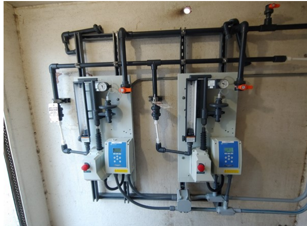
Week 87 – Ammonia system to the blend basin tied in and tested.
