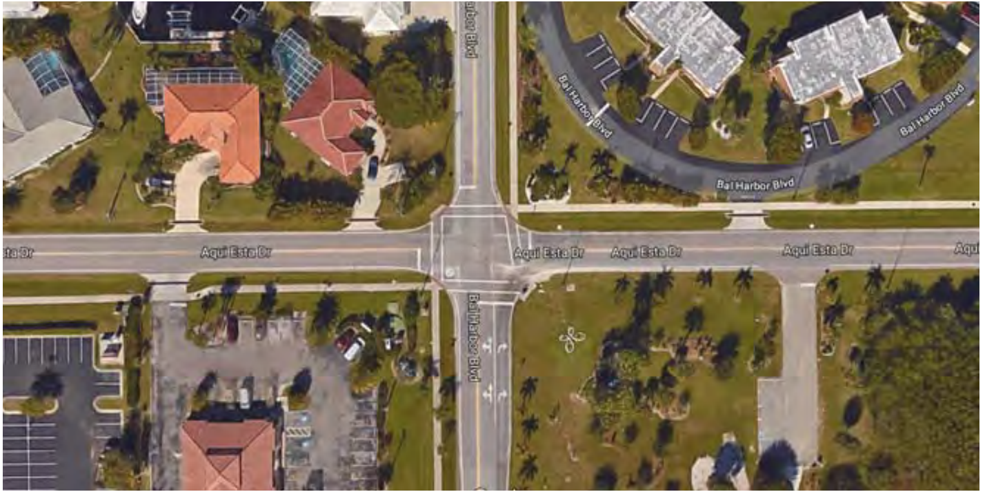
Existing Condition at Aqui Esta Drive and Bal Harbor Boulevard
