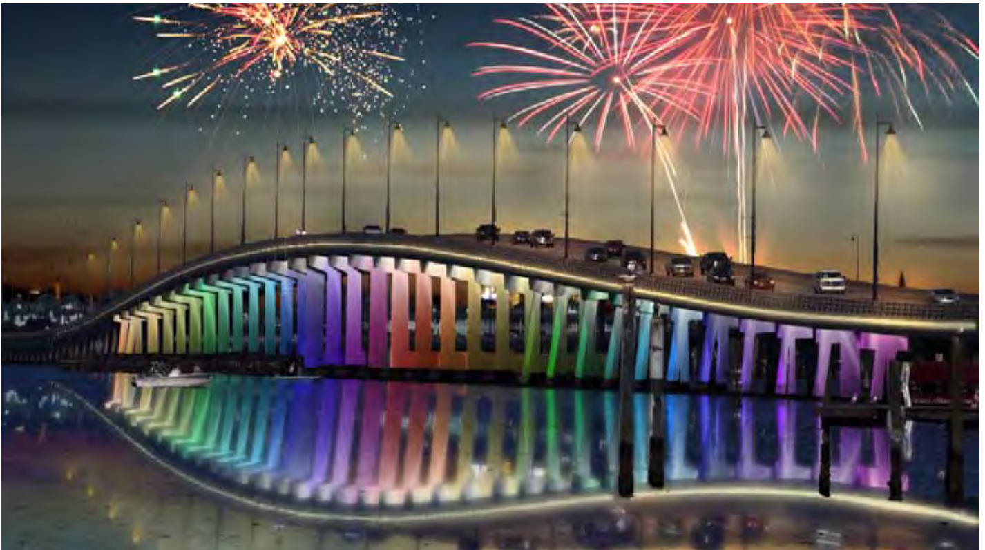
Gilchrist Bridge Lit Up with Rainbow LED Lighting for a Special Event
