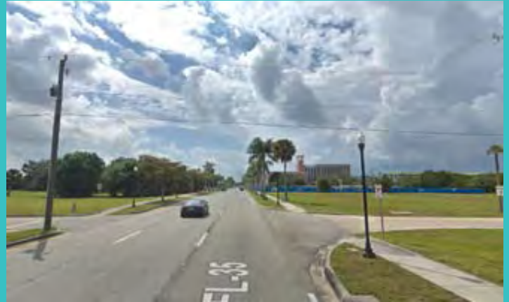
Existing conditions - Marion Ave
