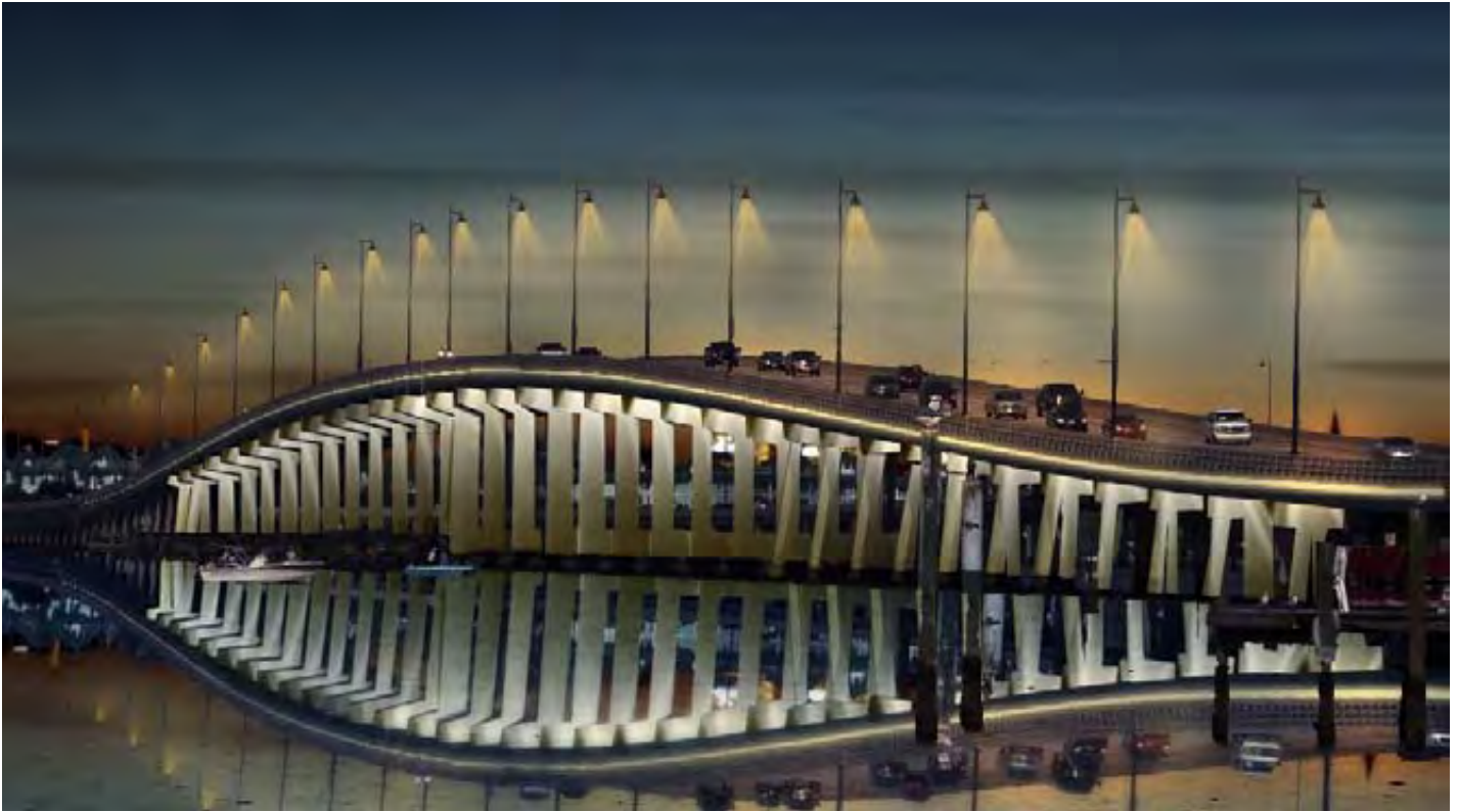
Gilchrist Bridge Lit Up with Soft White/Amber LED Lighting
