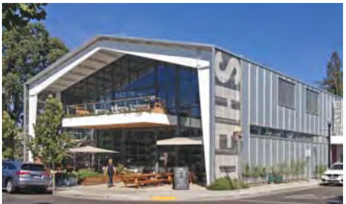
Prefabricated shed building, designed as a flexible space that could accommodate a market hall, small brewery, and events (Lincoln Lighthill Architect)
