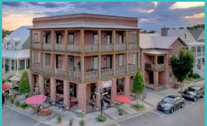
Hammond's Ferry a traditional neighborhood development (TND) in North Augusta, SC
