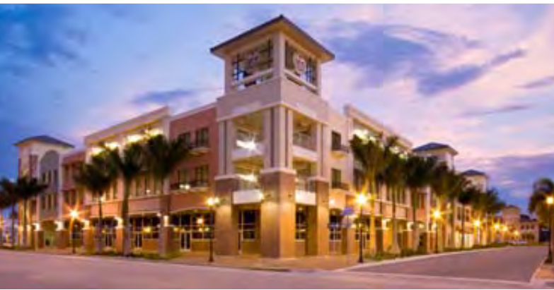
Herald Court Centre Project; Photo credit: City of Punta Gorda
