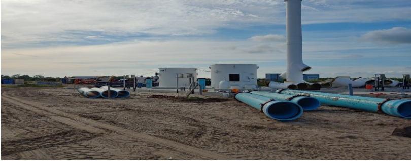
Degasifier being installed.
