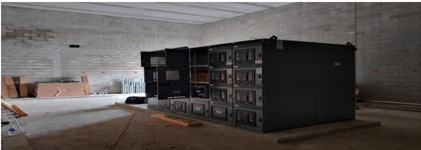
Switch gear placed.
