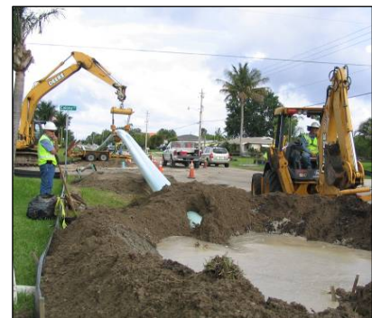
Installation of 1,160 LF Bore
