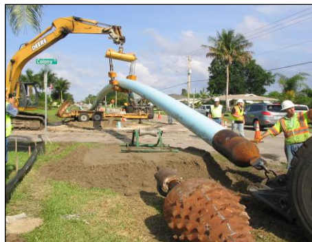
Elevated Entry to HDD
